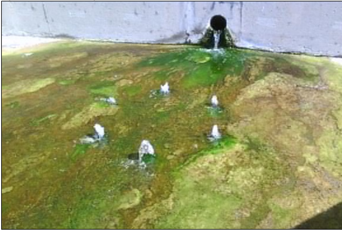
Figure 2. Manhole Exuding Groundwater into San Jose Creek
